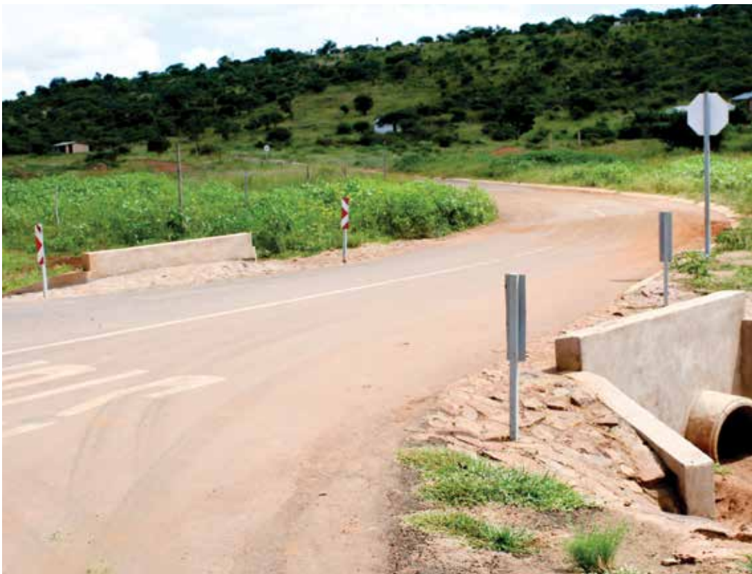
The newly completed 4.5-kilometre Ga Maepa Access Road
